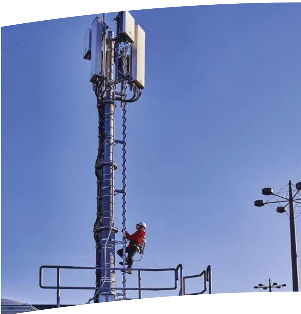
----- An engineer climbs a 5G network mast. Photo: Wolfram Schroll / Bloomberg via Getty Images
